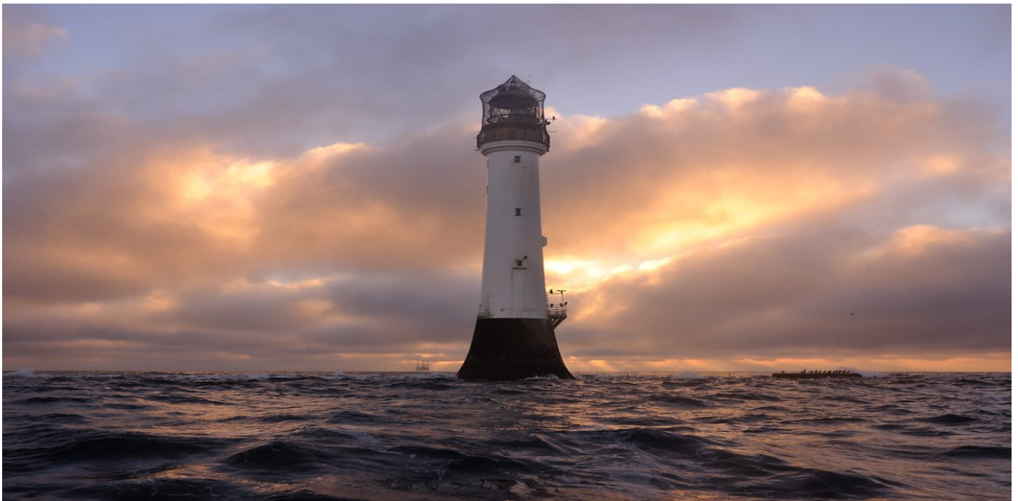
Bell Rock Lighthouse (1810), 12 miles off the coast of Angus – considered to be the most challenging of the lighthouses built by Robert Stevenson.
